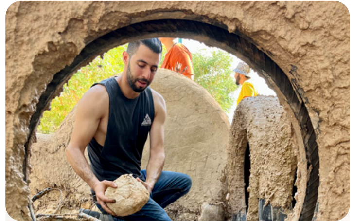
• Participants learned to make a mud mix and to apply it to walls. The above walls are made from mud, straw and tyres - notice the shape.
